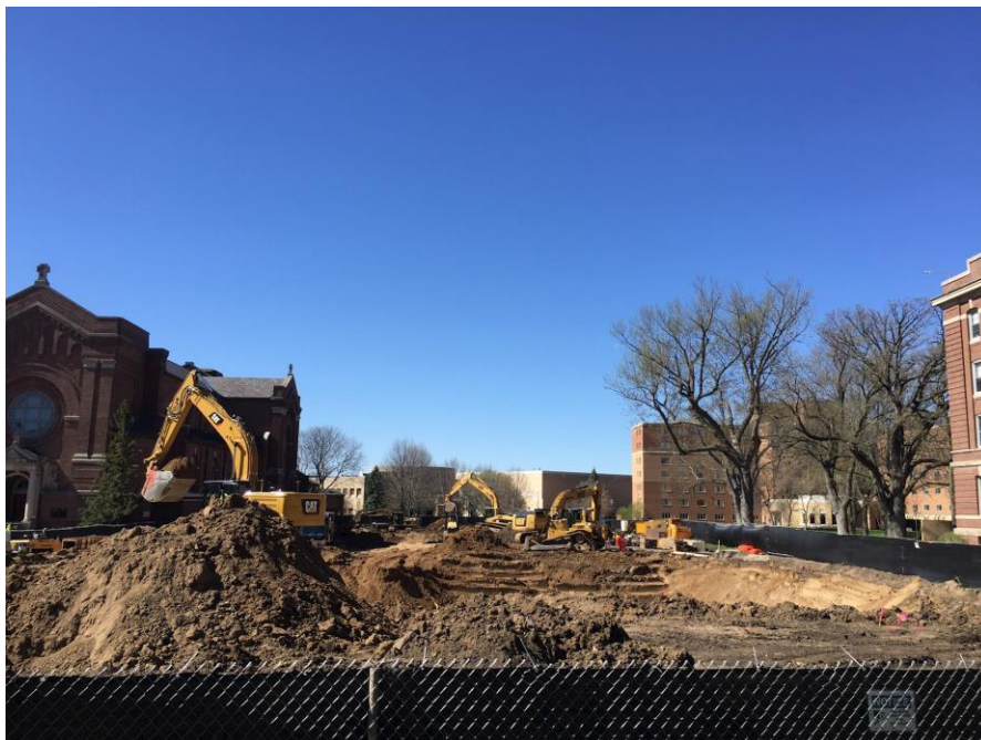
View of overall site excavation. Taken: April 26
