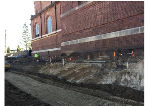
Start of original foundation underpinning. Taken: April 26, 2019
