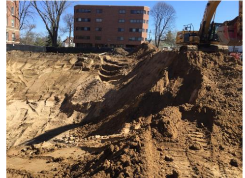
Looking at excavation for foundation. Taken: April 26, 2019
