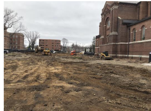
Looking North at Site. Taken: April 10, 2019
