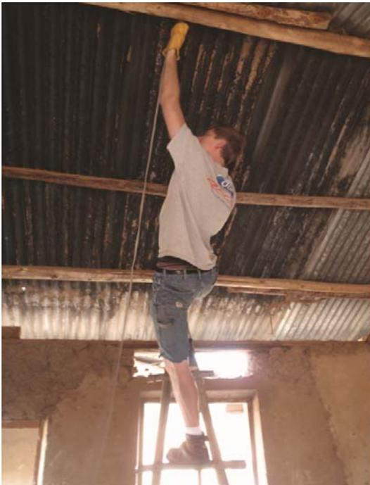
Figure 4: Photograph showing the installation of wiring within a dwelling.
